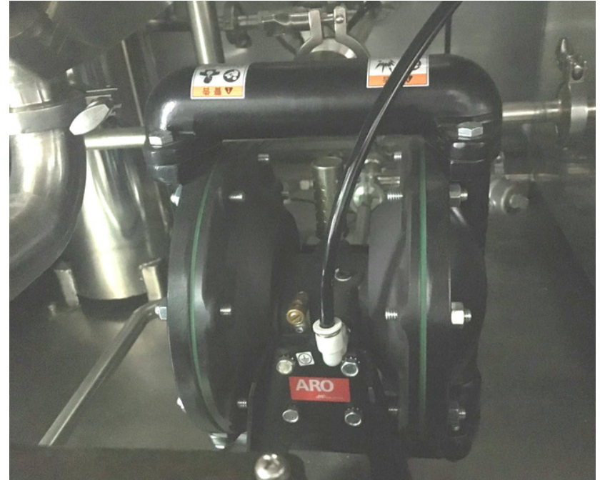
Ingersoll Rand air pump for liquid and water automatically adds and discharge.
